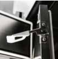
▲ Outer door latch with padlock panel
